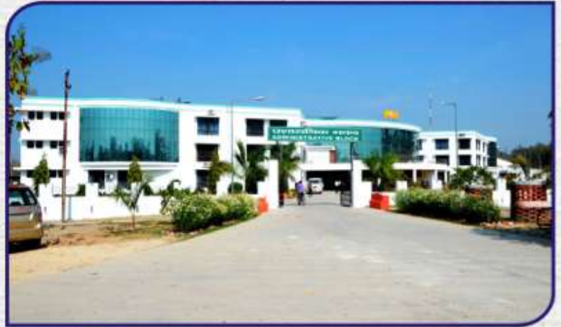
ADMINISTRATIVE BUILDING NDUA&T, FAIZABAD
